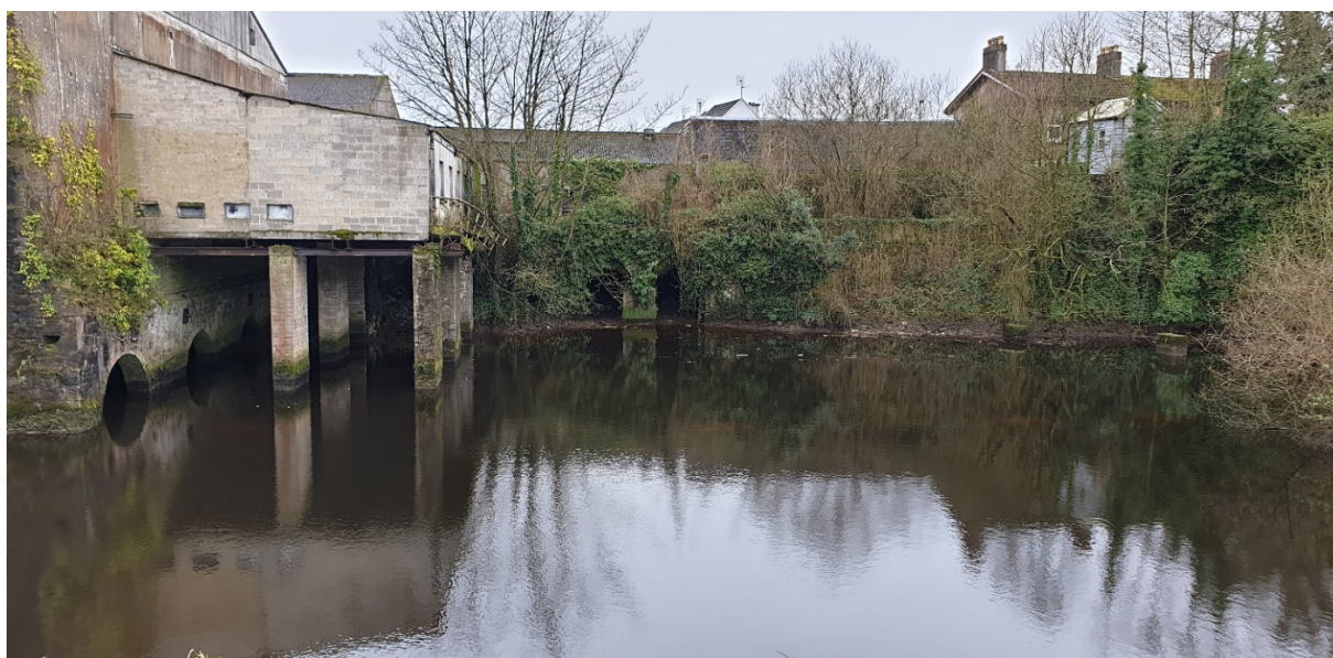
Figure 6: Existing reservoir in disused quarry on-site (February 2021)
