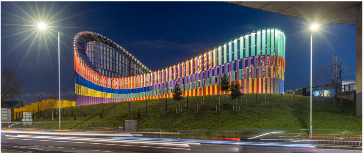
Figure 15: Brent Cross Town Substation © Arup
