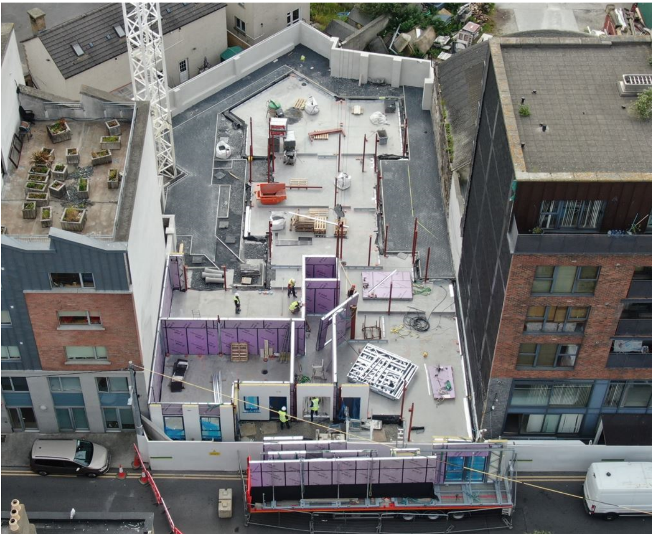
Figure 16: Pim Street Apartments: on-site assembly of 2D panels © Framespace
